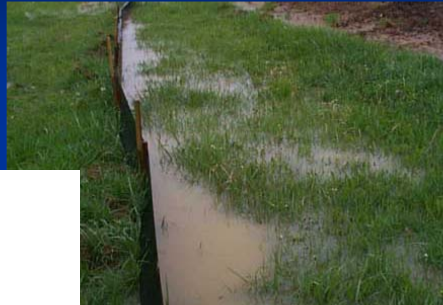
Silt Fence – Type A
